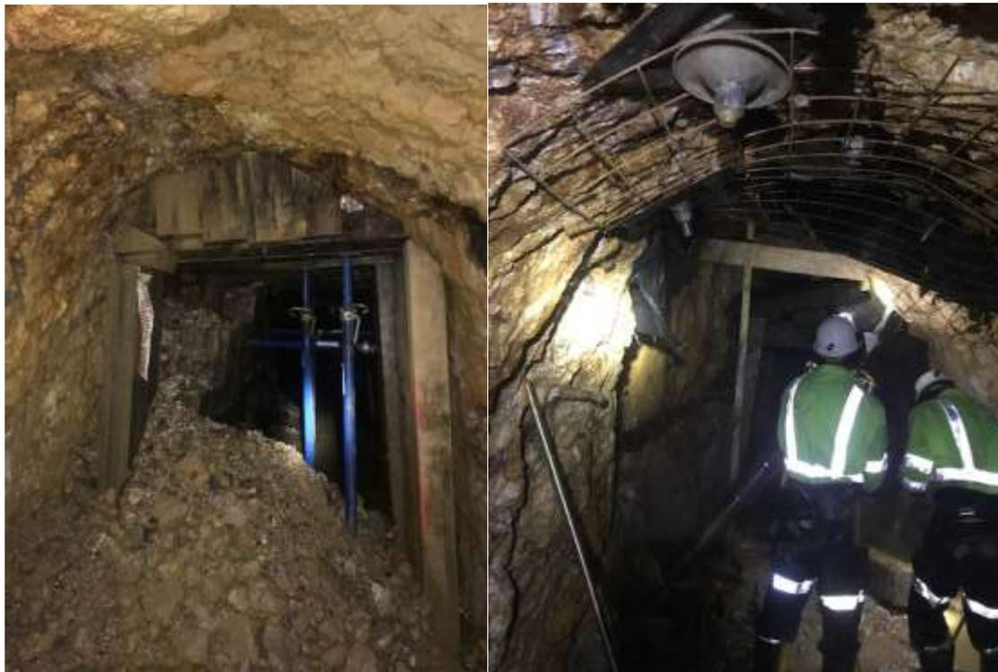
*Figure 2 – Before and after photos of rehabilitation work at the old ore pass*
