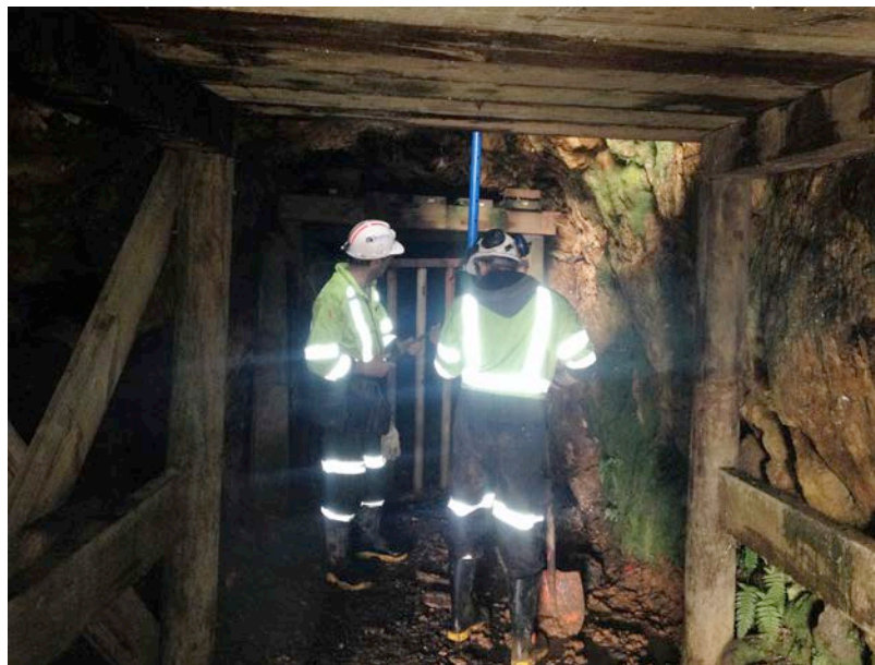
Figure 1 - Work in progress with support upgrades at the Talisman Project
