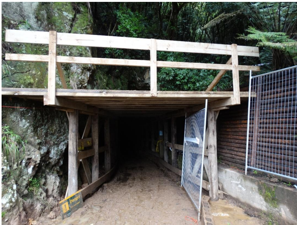
Portal entrance structure which will form part of the ventilation airlock
