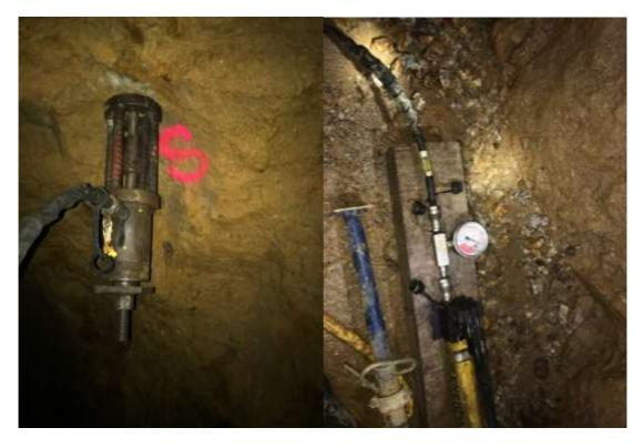
Figure 3 - Rock bolt undergoing pull tests after installation. A hydraulic jack is attached to the anchor and load applied to the bolt. This tests the performance of the contact between the bolt, the resin and the ground being supported.
