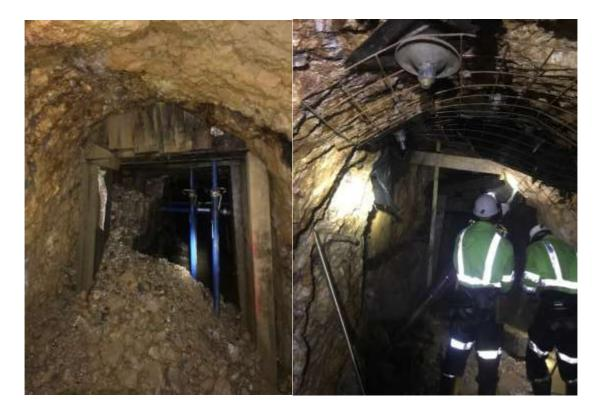
Figure 2 – Before and after photos of rehabilitation work at the old ore pass
