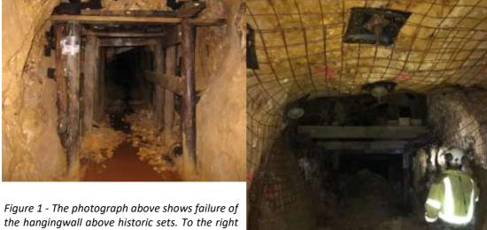
is a photo of the area after the sets had been removed and permanent support installed
