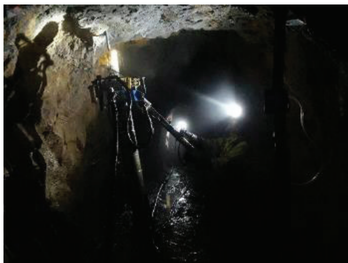
Figure 4 - installation of rock bolts in Keillors Crosscut
