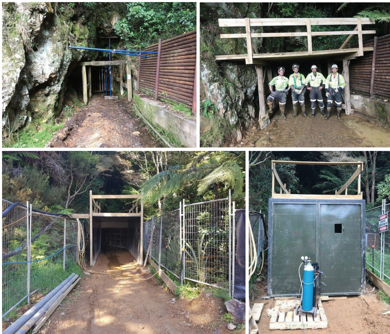
Figure 2 - photos showing reconstruction of portal support and the ventilation lock
